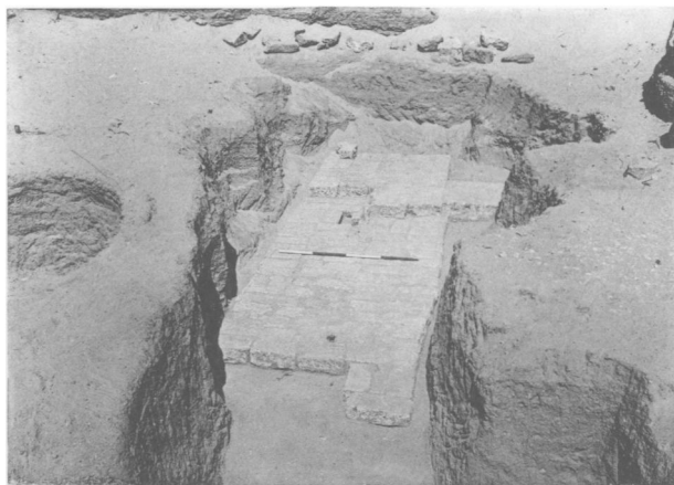
2. Site II. Foundations of early temple pylon and north wall running below the Temple of Taharqa
