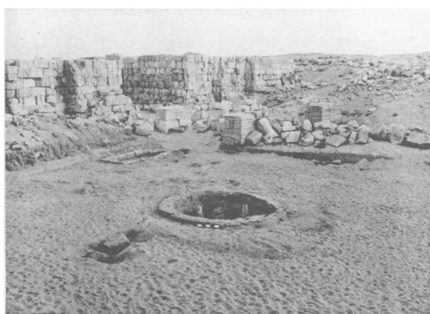
4. Sunk 'bed' with brick border, containing four amphorae, in front of north pylon tower of Temple of Taharqa. Looking south-east
